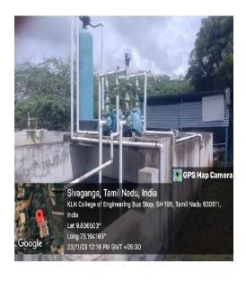
This plant is located nearer to the Ladies Hostel. Here drainage water is filtered and recycled by various water treatment processes. This recycled water is used for watering the plants in gardens.
